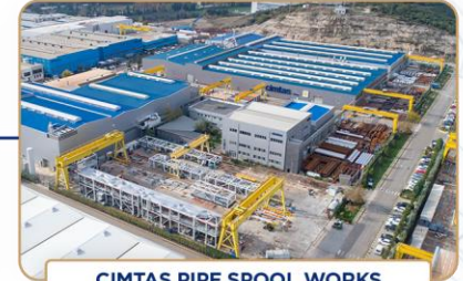
ÇİMTAŞ PIPE SPOOL WORKS
